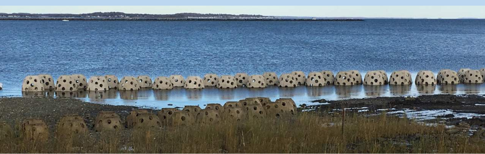
Reef balls. Photo credit: Connecticut Institute for Resilience & Climate Adaptation.
