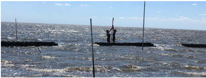
Photograph of Oyster Castle breakwaters, August 2019. Photo credit: Amy Bredes, Stevens Institute of Technology
